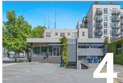
Pine Street Commercial 1313 Pine St, Seattle, WA 98122
