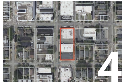
Roosevelt Redevelopment Site 6220 Roosevelt Way NE, 98115
